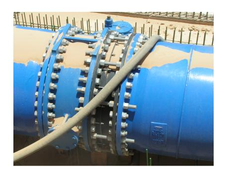
The double eccentric butterfly valve is well suited for water supply applications, used for their strength and resistance even at high pressure They are available in PN10, PN16, PN25 and PN40 up to a maximum of DN3600. Designed with tilted and fixed disc for extended service life and easy operation.
