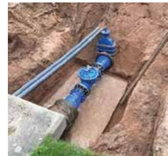
Automatic Control Valve Series 859 Installation
